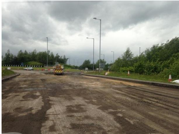
This week base course and binder has been laid between East Common Lane - the Wishing Well roundabout and between the swing bridge - northern layby averaging 1100 tonnes a day.
