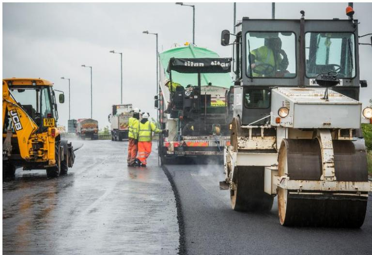
The heavy plant / machinery continues to plane out to a depth of 270mm in excess of 1000 tonnes of planings a day are being transported off site by a convoy of wagons.
