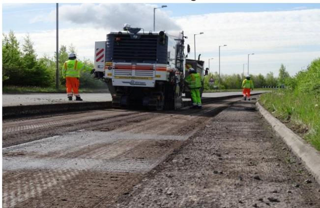
The plant / machinery has continued planing out to a depth of 270mm. This week over 4000 tonnes of planings have been transported off site.
